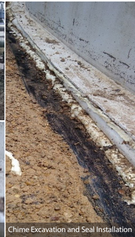
Chime Excavation and Seal Installation
