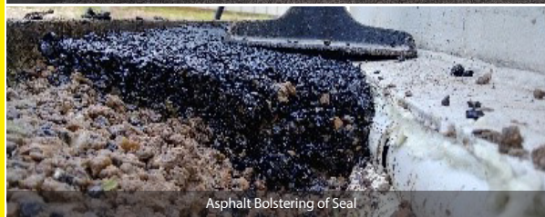
Asphalt Bolstering of Seal
