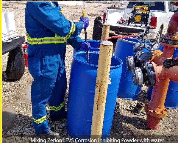
Mixing Zerion® FVS Corrosion Inhibiting Powder with Water
