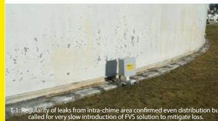
T-1: Deteriorating concrete and extremely heavy caulk needed in the intra-chime area, calls into question the over-all integrity of these tanks.
