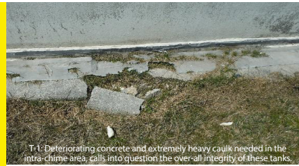
T-1: Deteriorating concrete and extremely heavy caulk needed in the intra-chime area, calls into question the over-all integrity of these tanks.
