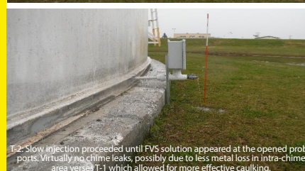
T-2: Setting up on the dike wall allowed for low pressure (nearly gravity feed) conditions. Only the injection ports were needed to evenly introduce the FVS solution. (unlike tank T-1)
