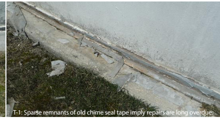
T-1: Sparse remnants of old chime seal tape imply repairs are long overdue.
