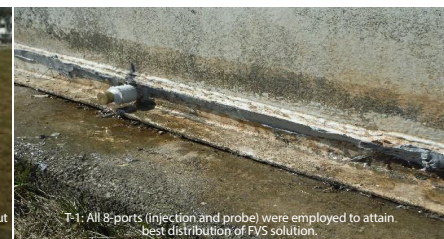
T-1: Sparse remnants of old chime seal tape imply repairs are long overdue.
