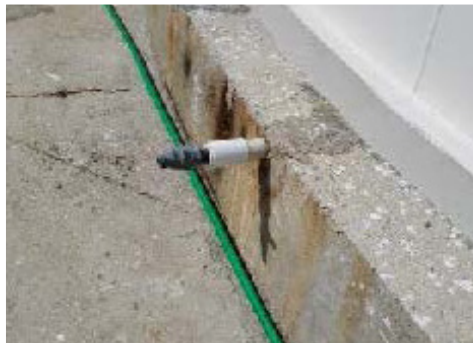
5. INSTALLATION OF INJECTION BALL VALVES
