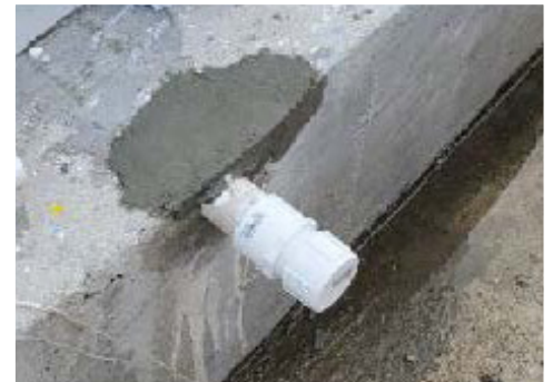
9. GROUT REPAIR
