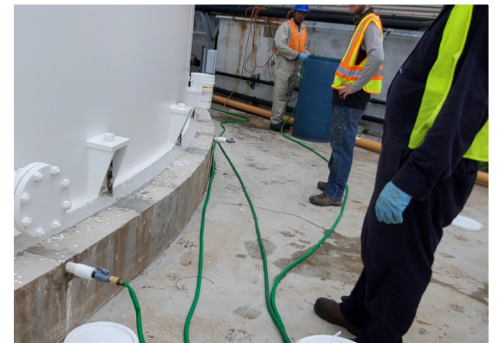
6. VCI SLURRY INJECTION
