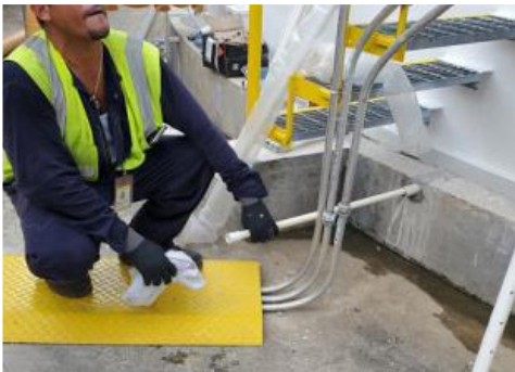
7. INSTALLATION OF PIPES WITH VCI SLEEVES
