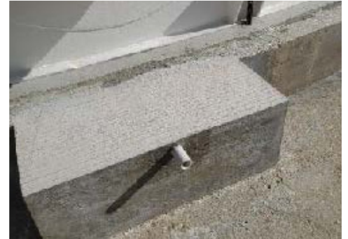
3. TRENCH VCI PORT
