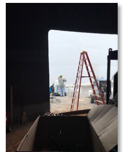
FIGURE 4: MIXING SITE AND DOORWAY
