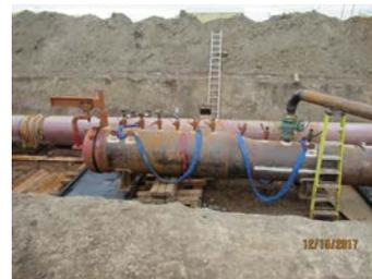
*This pipe is where the back pig is within the pipe. The valves on top of the pipe are used to add backpressure to pressure up battering ram from within.*
