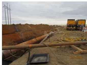
*Air compressors are used to force air through hoses into the pipeline to push the pigs throughout the length of the pipeline.*
