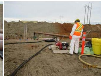
*The Zerion FVS slurry mixture is pumped out of the vacuum truck through suction hoses into the pipeline to fill the pipe in the trench with slurry.*
