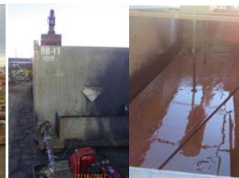
*A frac tank was used to hold the mass amount of excess Zerion FVS slurry from the end of the pipe after the pigs traveled through was then suctioned into the initial vacuum tank truck.*
