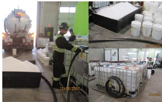
*Vacuuming Water and Propylene Glycol from totes and Zerion FVS Powder from bin into vacuum truck.*
