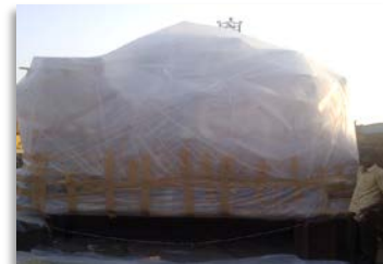
After Final Wrapping of Panel Boards
