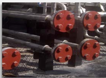
WGC Condition After Cleaning
