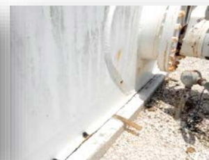
Installation of UT Scan Ports and Coupon Ports
