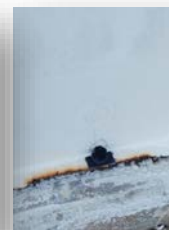
Installation of UT Scan Ports on Problematic Areas of Tank Chime
