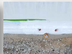
Complete Installation of Coupons and Inhibitor Sleeves
