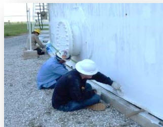
Preparation of the Tank Chime
