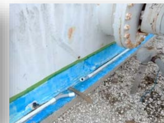
Installation of the “Chime Ring Dry” IDS PVS Pipes
