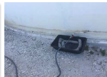
2. INJECTION PORT SETUP
