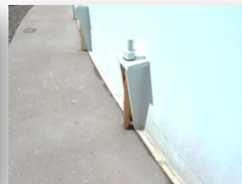
Cleaned and Marked Chime Area
