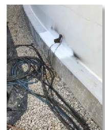
6. PATCH TO CHIME SEAL W/FLEX SEAL SPRAY
