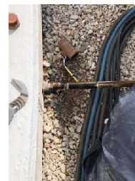
3. SW PORT USED FOR SLURRY INJECTION
