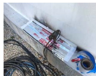
5. PATCH TO CHIME SEAL
