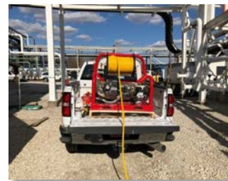
1. JRGO LLC PUMPING SYSTEM
