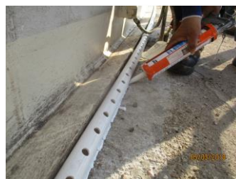
1. CHIME RING IDS PIPING SYSTEM
