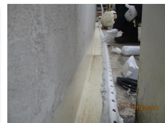
2. APPL. OF SEALANT PASTE
