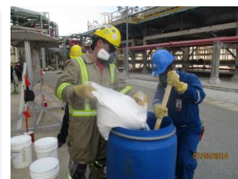
4. MIX. OF CORROSION INHIBITOR SLURRY
