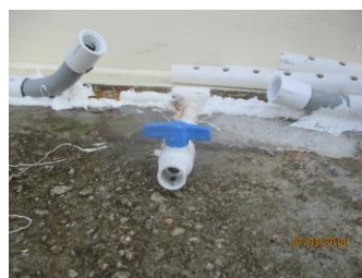
3. INSTALLED DRAIN PORT ASSEMBLY
