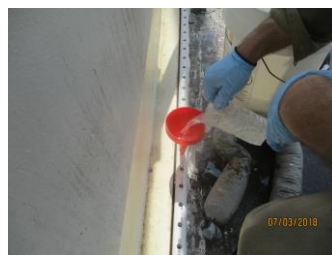
5. APPL. OF CORROSION INHIBITOR SLURRY
