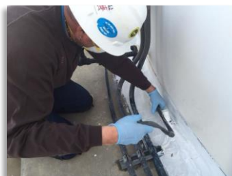
Inhibitor sleeves installation.
