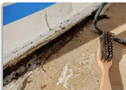
Preparation of the concrete tank chime and surfaces.
