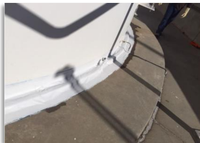
1 st coat of maximum stretch application.
