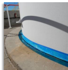
Application of the 1 st of 2 coats of blue max primer.
