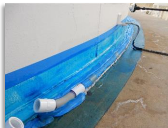
Installation of the "Chime Ring Dry" IDS PVC Pipes
