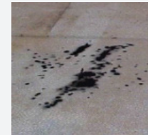
Holes in the roof of an AST
