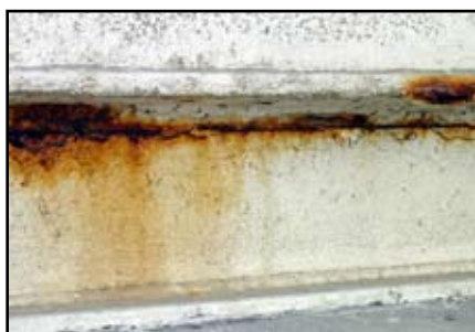
CORROSION DAMAGE ON THE UPPER BOTTOM PLATES OF THE ABOVEGROUND STORAGE TANK
