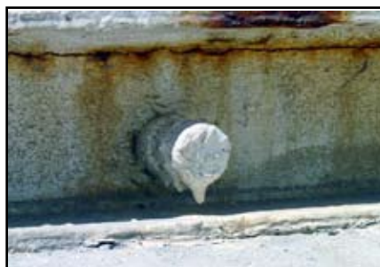
CORROSION DAMAGE ON THE UPPER BOTTOM PLATES OF THE ABOVEGROUND STORAGE TANK
