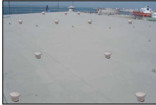
VIEW OF DISPENSER ON TOP OF 54m DIAMETER TANK
